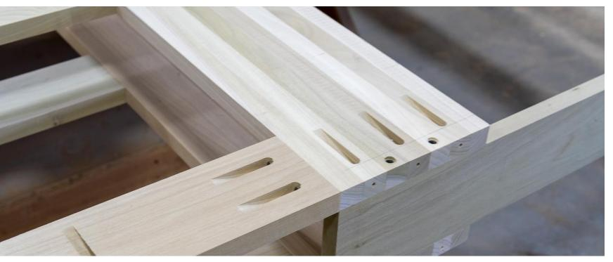
Recessed joinery ensures tight fit and finish and ensures drywall sits flush on cross members
